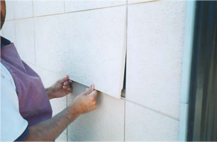
J. The panel is replaced and the watertightness of the CAREA system preserved.
