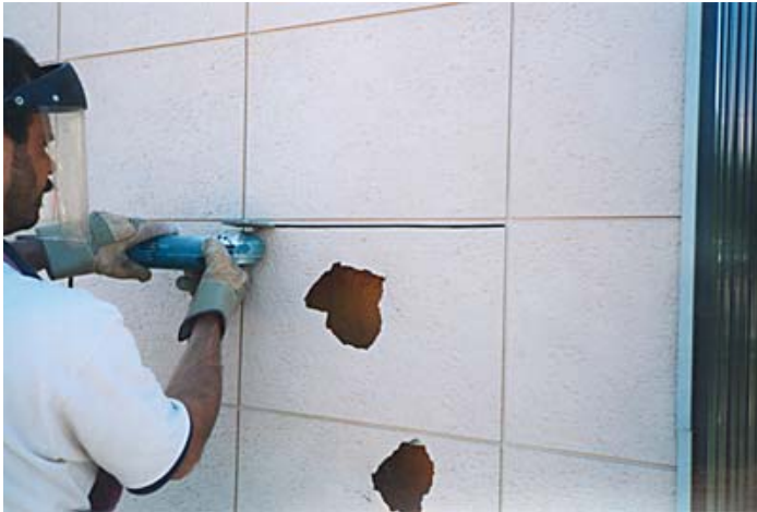
A. Perform horizontal cut 1 cm (1/2") below top joint of broken panel.
