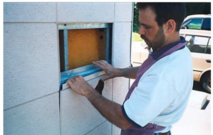
E. The wall is ready to receive the replacement panel.
