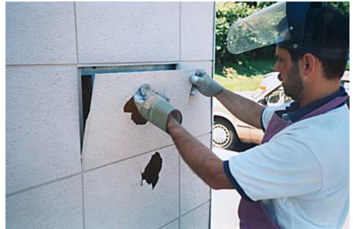
C. By lifting upper right corner, remove broken panel.
