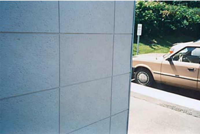
J. The panel is replaced and the watertightness of the CAREA system preserved.
